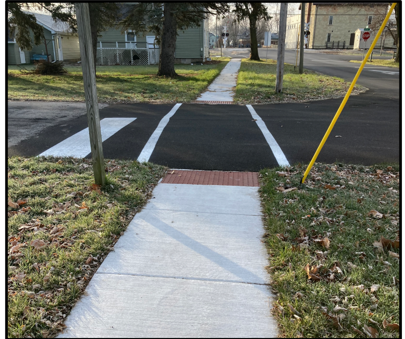
The above curb ramps and depressed corners consist of detectable warnings and geometric slopes that are “compliant” with the current ADA standards. All future construction will meet the current ADA standards.
