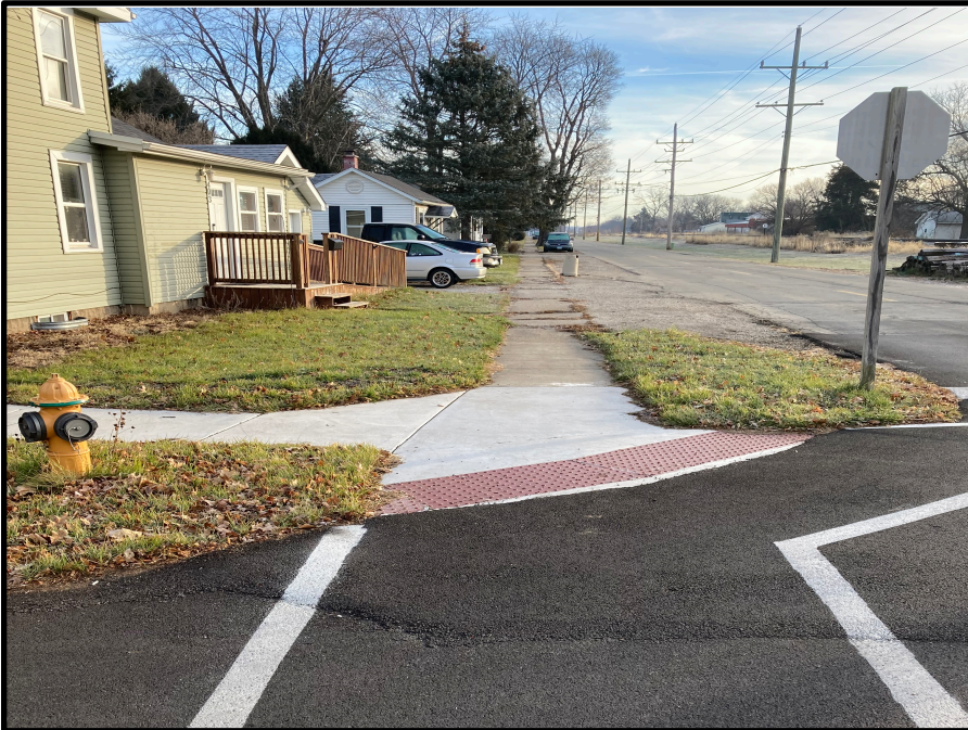
The above curb ramps and depressed corners consist of detectable warnings and geometric slopes that are “compliant” with the current ADA standards. All future construction will meet the current ADA standards.
